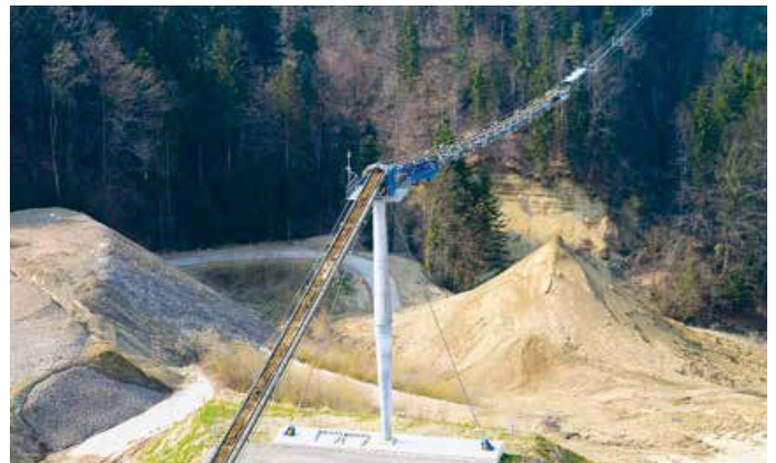
2016 The RopeCon® installation that has been operating at the Tüfentobel waste tip near St. Gallen (CHE) since 2005 is extended by a second RopeCon® incorporated directly within the rope span. Material transfer takes place at a height of roughly 20 m.
