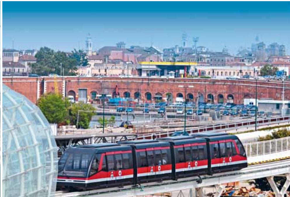
CABLE Liner Shuttle – Venezia, ITA
