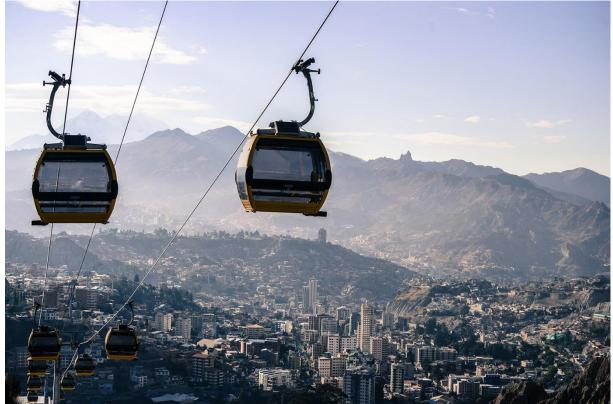
The detachable gondola lift has proven itself in La Paz, the same ropeway system will now be built in Bogotá.
