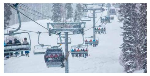
The Centennial Express Lift provides a 35 percent increase in transport capacity over the old lift and can carry 3,400 passengers an hour.
