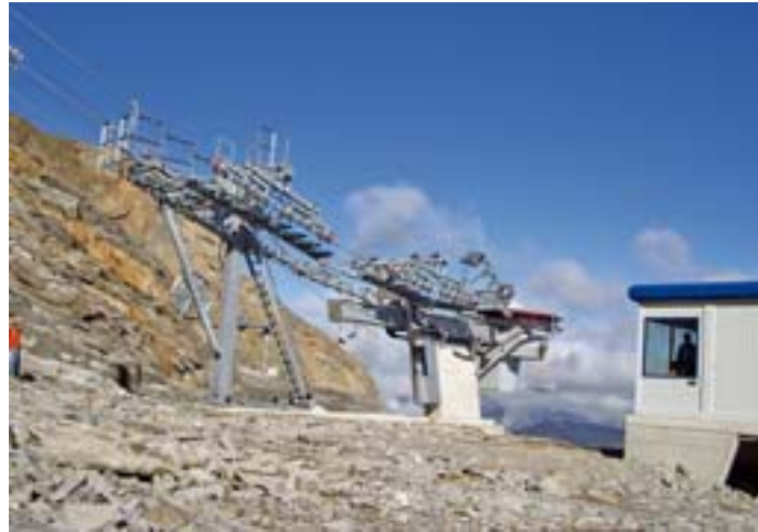
Bottom terminal of Kaserer 1 below the Hintertux Glacier at an altitude of 2705 m: at the front the mast for guy rope tensioning, behind it the drive with 230 kW DC motor and hydraulically operated platform for relocating the grips.
