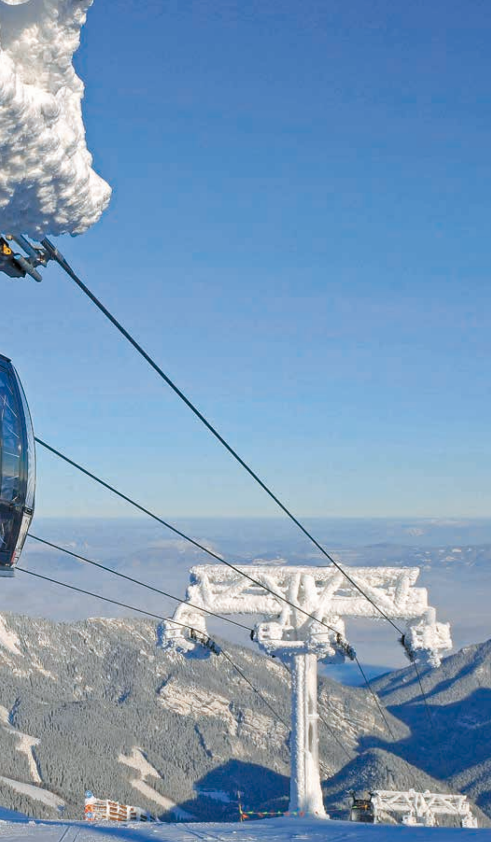
Unique technical feature: The twisted curve tower structure on the Krupová surface lift
