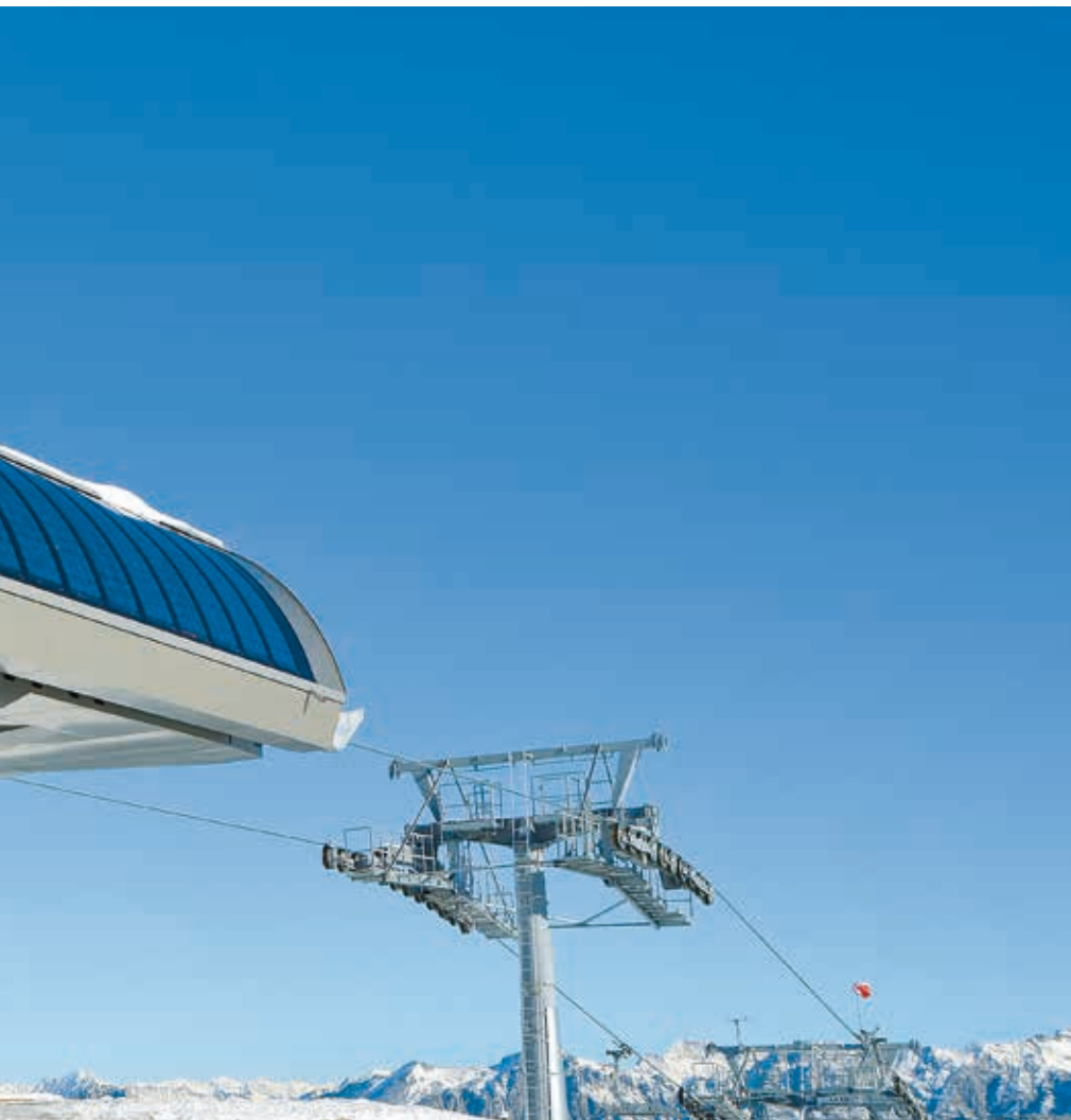
Photovoltaic modules are also integrated into the bottom station building.
