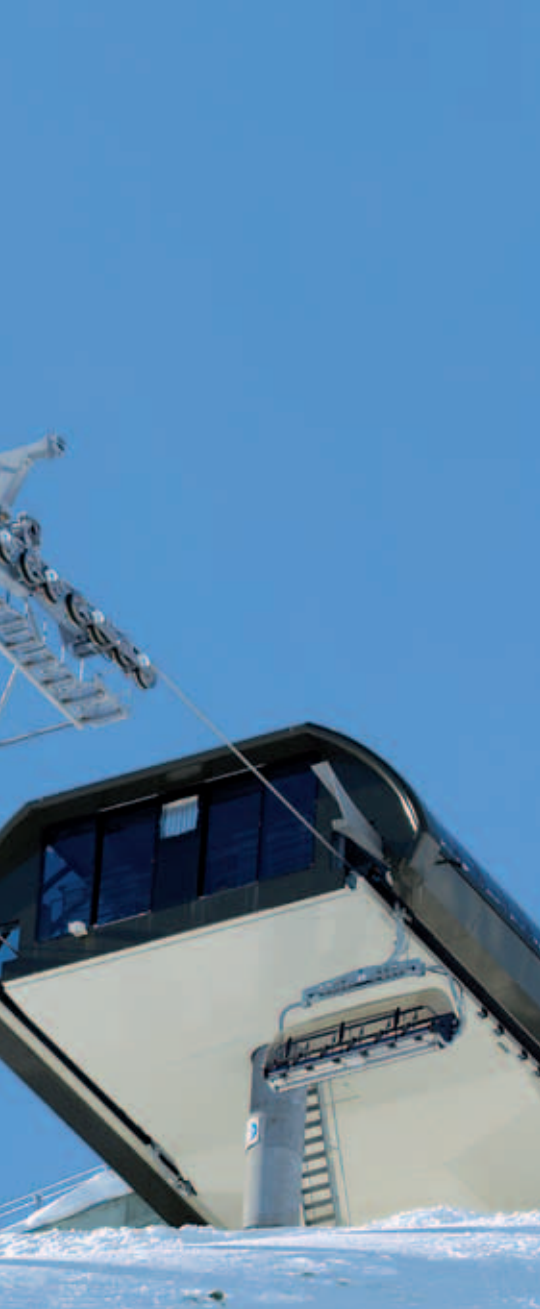
The top station at an altitude of 2,820m was partly built into the mountain to minimize the visual impact on the landscape.
