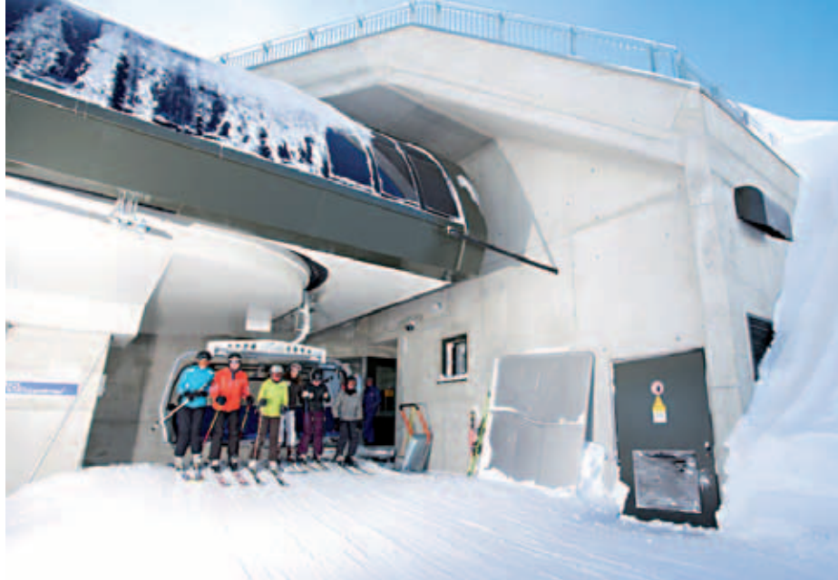
The top station at an altitude of 2,820m was partly built into the mountain to minimize the visual impact on the landscape.
